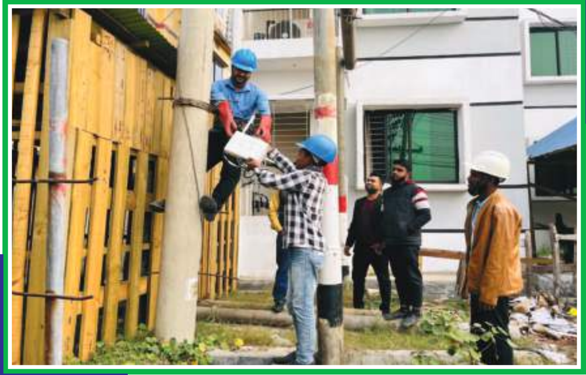
DCU Installation Work at Dhaka PBS-4
