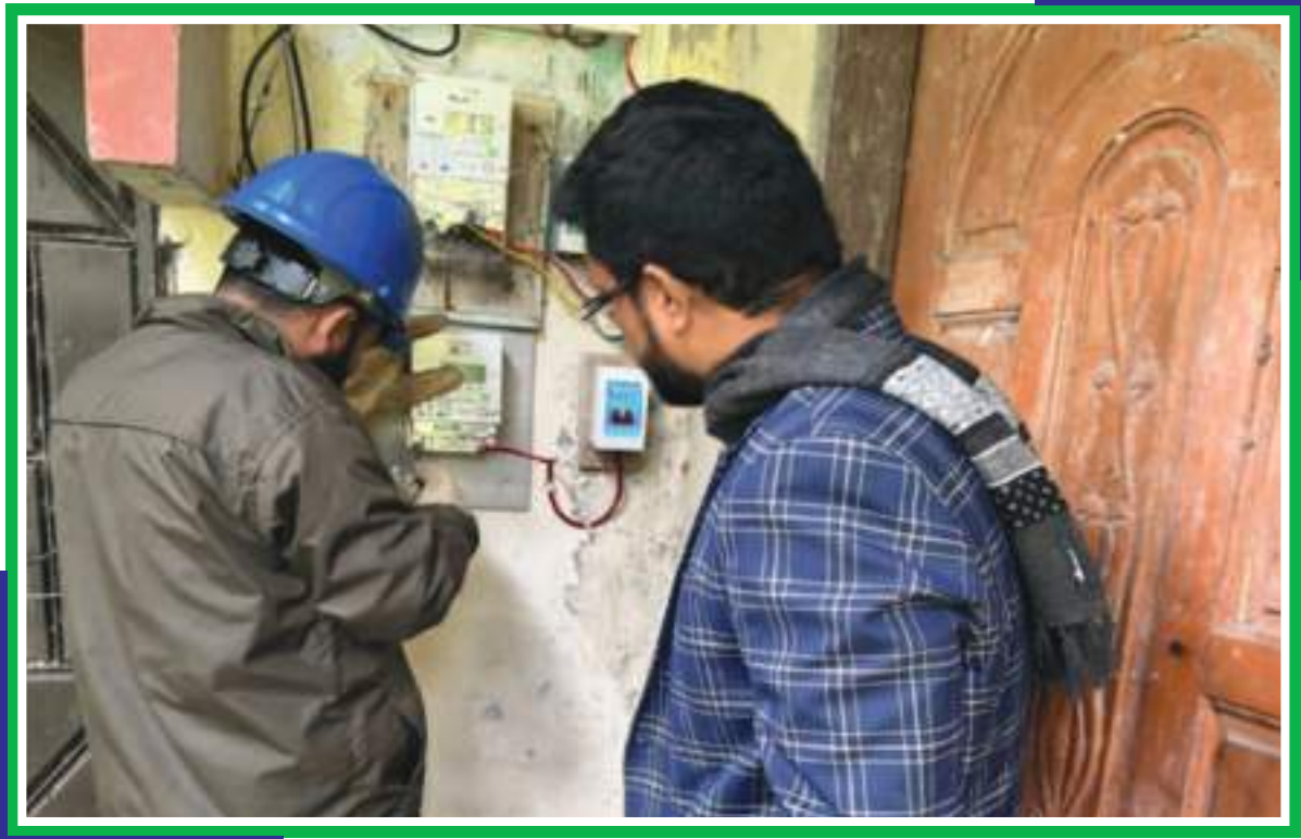
SPPM Installation Work at Dhaka PBS-4
